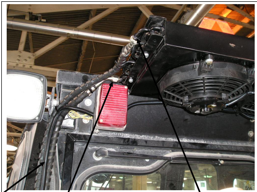
Power wire from relay.
